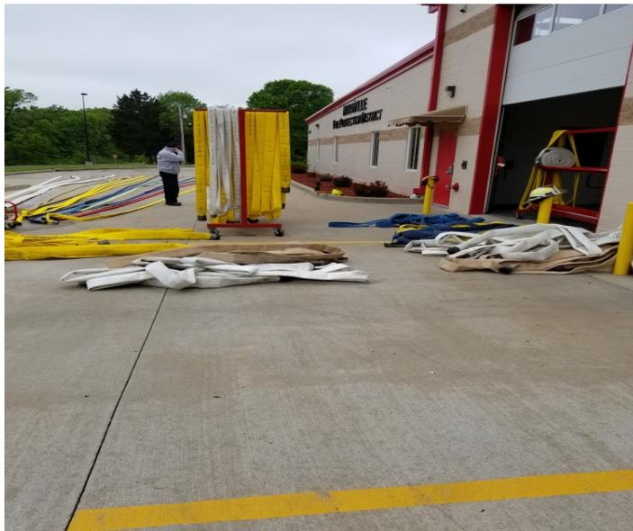
Hose testing is a very important component, as it not only verifies that the fire hose is capable of handling the water pressure and the water volume necessary to extinguish fires, it certifies that annual inspection and maintenance to the hose is being accomplished on a regular schedule. In addition, the hose testing program that has been instituted creates a positive effect on our I.S.O. review that establishes the insurance rating and premiums for all Mapaville residents.
